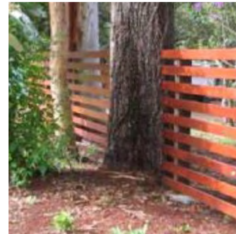
Figure 4.1.2. Fences incorporating trees and of slatted design provide ideal movement solutions for fence permeability to koalas.
