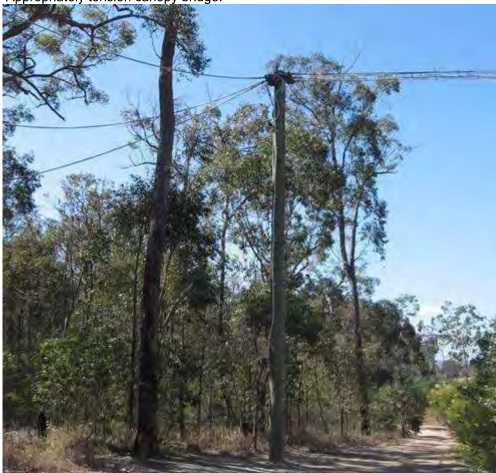
Figure 6.4.3 Canopy bridge at Compton Road, Brisbane. Bridge is connected to the surrounding environment by ropes (Robinson-Wolrath 2007).
