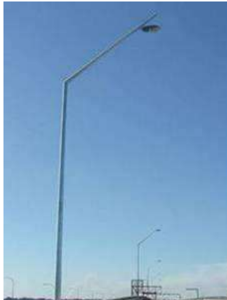
Figure 6.13.2 Light pole designed to deter roosting opportunities
