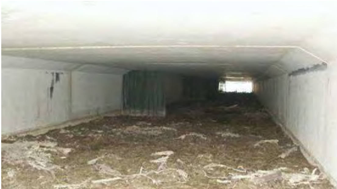
Figure 6.6.7 a) Frog culvert at Tugun Bypass (Robinson-Wolrath 2007). b) Frog culvert at Tugun Bypass with shade cloth installed to provide amphibian refuge (Robinson-Wolrath 2007).
