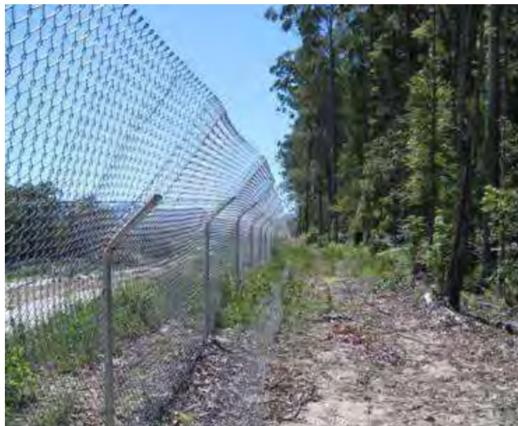
Figure 6.11.4 Plastic strips at the base of fauna exclusion fencing can be used to prevent movement of reptiles into the road corridor (Scott 2007).
