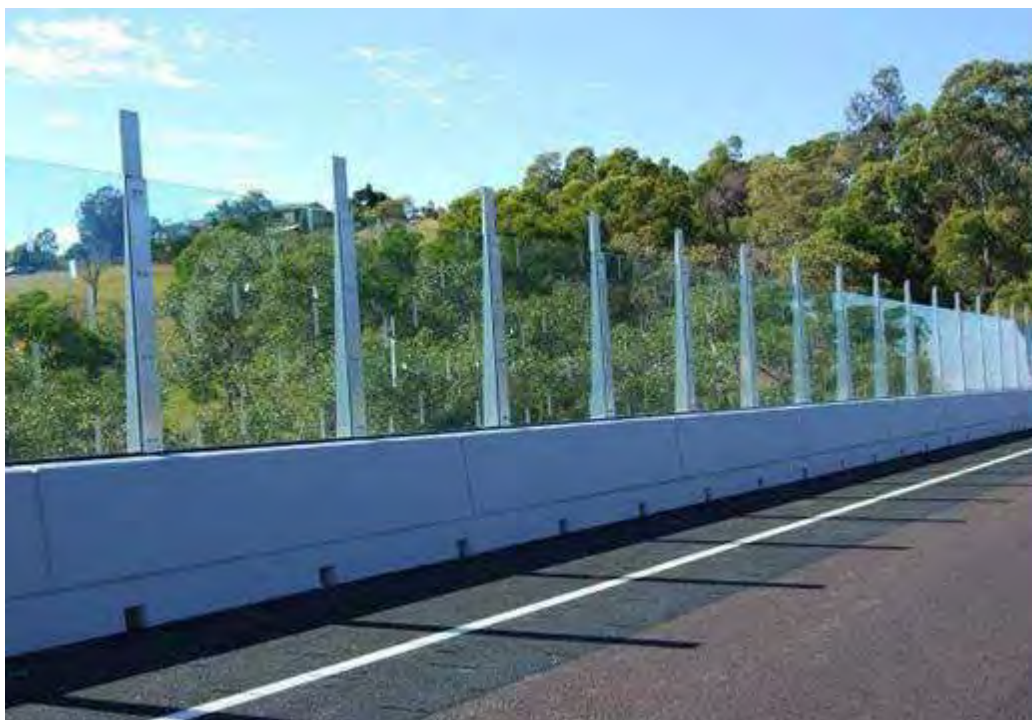
Figure 6.18.7 Transparent noise wall with etchings to reduce bird strike along the Tugun Bypass (Taylor 2008).
