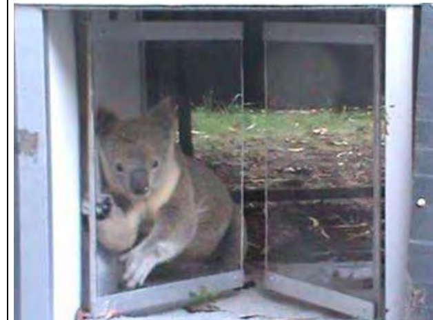
Figure 4.3.17. (photo: Jonathan Hanger) Perspex gates with a spring balanced/counter lever design will wield to gentle pressure of a koala pushing through the gate flaps in one direction but will not allow a koala to push open the gates to access the road corridor.
