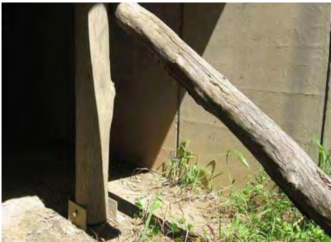
Figure 6.6.13 Lead up pole to a horizontal log used to traverse the culvert at a safe height (Robinson-Wolrath 2008).
