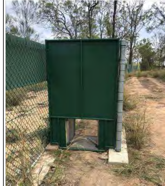
Figure 4.3.16. (photo: Jonathan Hanger) A koala escape gate is fitted along fencing to provide one-way access out of the road corridor.
