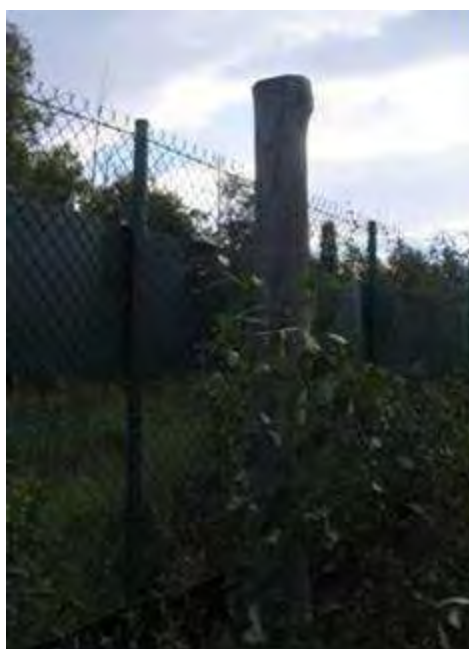
Figure 6.5.6 Escape pole at Compton Road, Brisbane. Note: Koalas must be assisted to return to vegetative side of fence.
