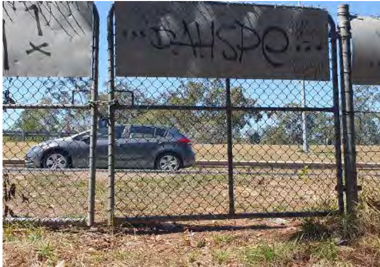
Figure 4.2.7. (photo D de Villiers) Poorly designed gates provide avenues for koala egress to the road corridor (gaps are shown between and under the gates).
