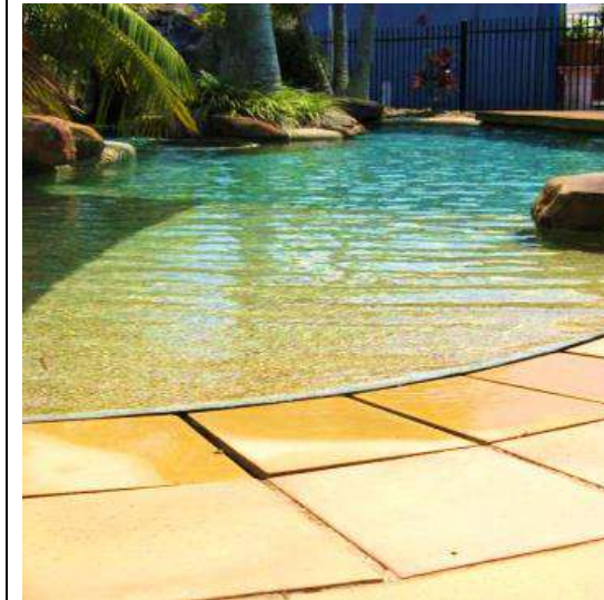
Figure 4.6.2. (photo: D de Villiers) Pools with lagoon-style exit points allow koalas to easily exit the pool.
