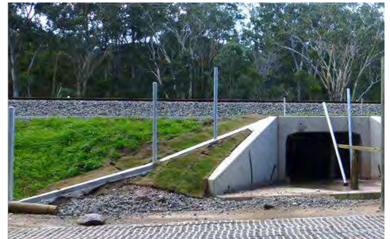
Figure 4.3.13. (photo D de Villiers) Koala exclusion fencing constructed along a rail line. Without barrier fencing, koalas will likely walk across the rail line and avoid the dedicated fauna crossing point/culvert. Fencing completed below.
