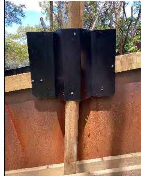
Figure 4.2.4. (photo David Fleay Wildlife Park) Fencing supports fitted with a 'koala shield' prevents koalas climbing the support.
