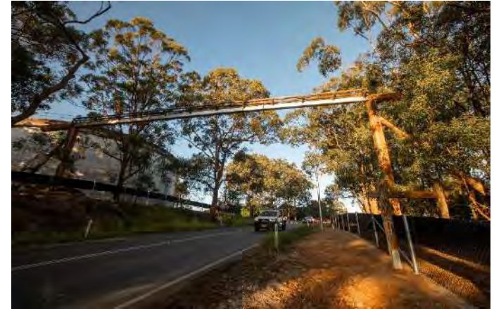
Figure 4.3.10 a. (photo: Brisbane City Council). An overpass links habitat on either side of Boundary Road, designed for koalas and other fauna
