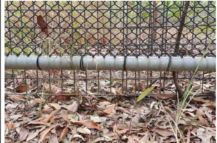
Figure 4.2.6. (photo D de Villiers) Fencing can be retrofitted with additional wire cover gaps under koala proof fencing where the ground is undulating.
