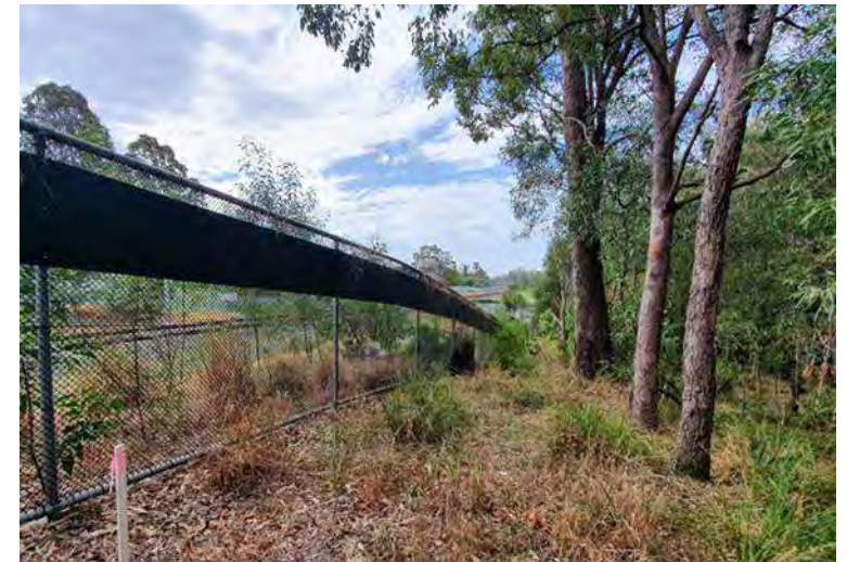
Figure 4.2.5. (photo D de Villiers) Unclimbable metal sheeting should be fitted to fencing over 1.5 m at a height that is comfortable for a koala to jump to the ground. All vegetation within 3m of the fence has been removed.
