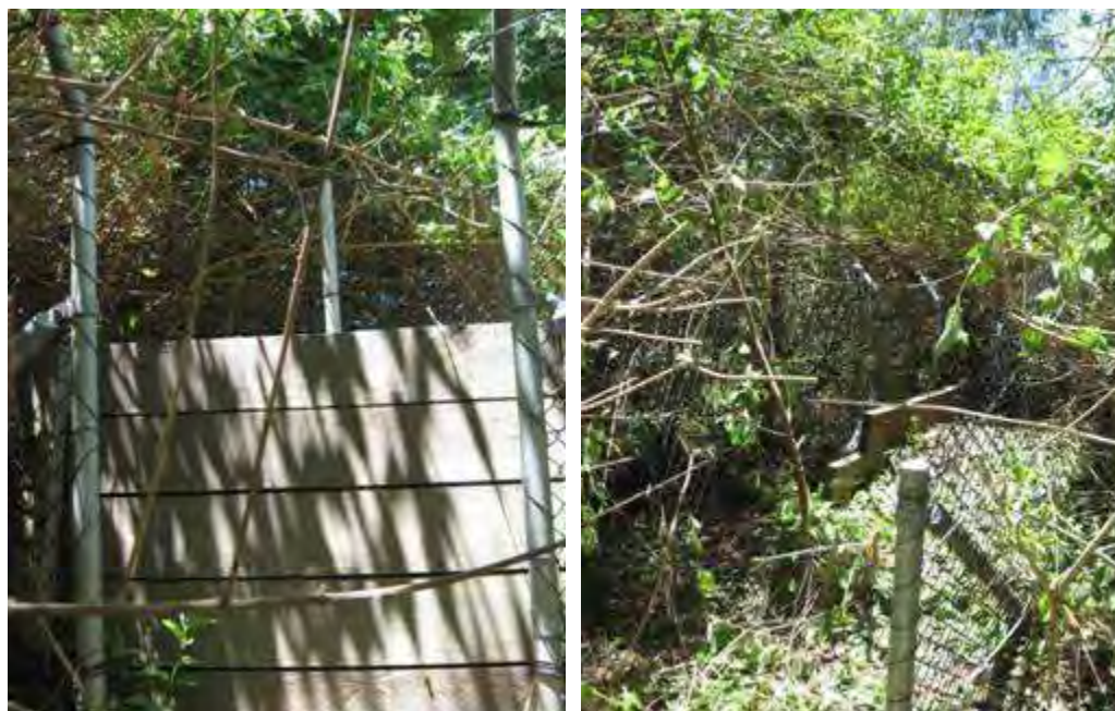
Figure 6.11.6 One-way fence to allow koalas to escape from the road corridor. a) Photo taken from the drop-off side of a one-way fence located at Yelgun to Chinderah section of the Pacific Motorway (NSW Roads and Traffic Authority). b) The ramp leading up to the drop-off side of the fence.
