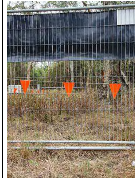
Figure 4.4.3.(photo D de Villiers) Temporary fencing is typically secured on footings with panels raised off the ground. This design allows egress of fauna into unsafe areas during clearing operations or in the construction zone.
