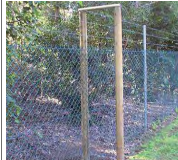
Figure 4.1.4. A wooden bridge over security fencing designed to facilitate the safe movement over the fence and barbed wire by koalas but effectiveness is not well established.
