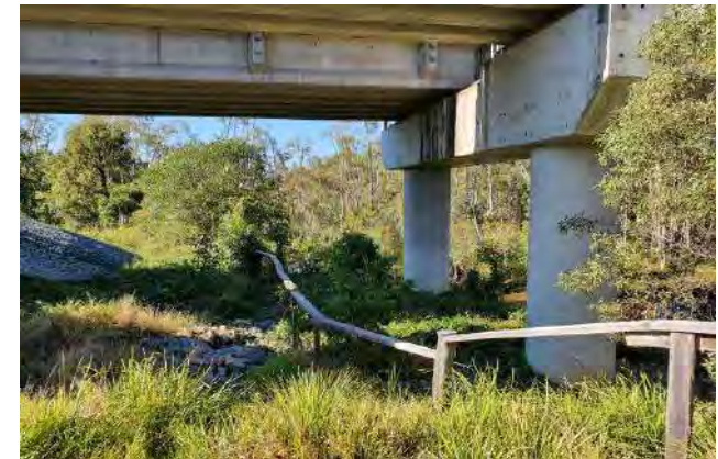
Figure 4.3.11 (photo D de Villiers) Under-bridge crossing point for wildlife, with wide buffer to bridge footings that can accommodate fauna furniture to assist with movements and predator avoidance.
